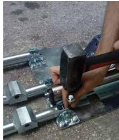
**Figure 10 - Anchor placement**
