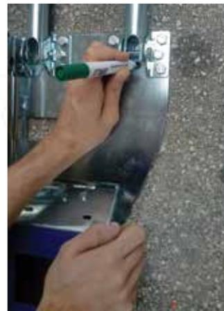
Figure 8 - Marking drilling spots
